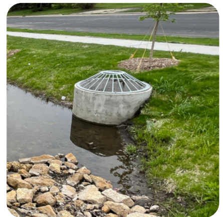
A riser pipe with trash rack
