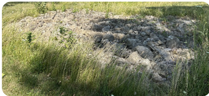
A riprap reinforced overflow spillway with minor vegetation growth
