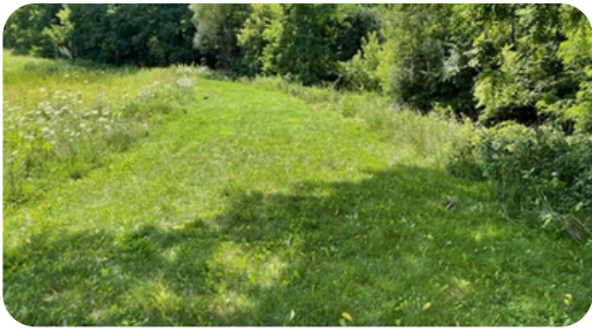
The berm of an infiltration basin with tree growth on the side slopes
