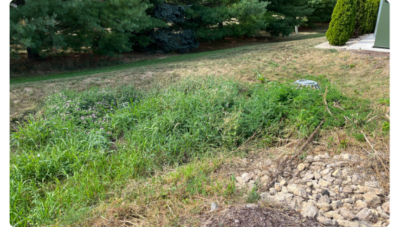
A bioretention basin that has not been properly maintained. Weeds have taken over and covered the outlet structure.
