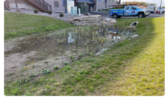
A bioretention basin that has remained wet due to clogging and overwatering, preventing proper vegetation growth.
